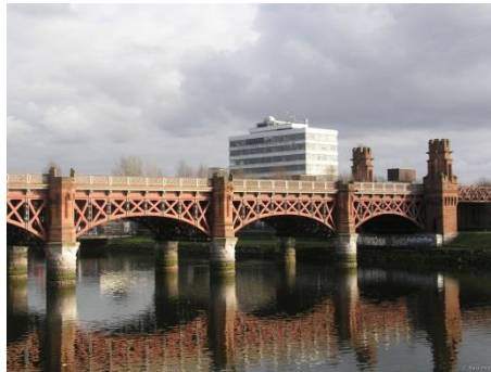
Union Railway Bridge 259283 664510
